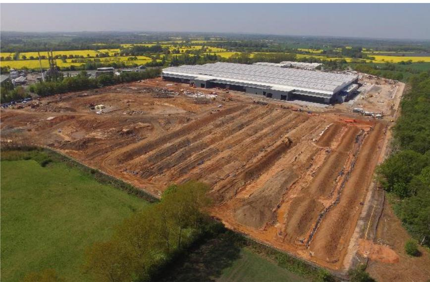
We worked with Hydrock Consultants to develop a robust and cost effective Remediation Strategy and implemented it as part of the redevelopment programme. This involved working closely with Readie Construction and key subcontractors (piling, groundworks and utilities) to manage the site's shallow water table and phase the remediation works efficiently, enabling the successful completion of a 450,000 sq ft manufacturing facility.
